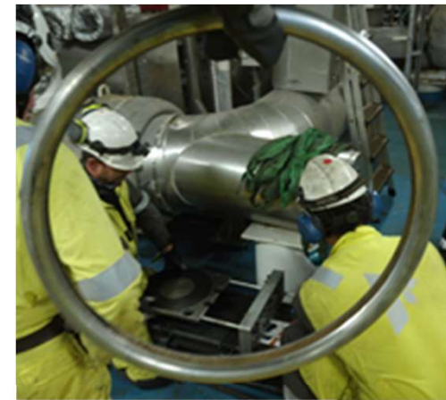
Gasket removed from live 150 HC Gas system
